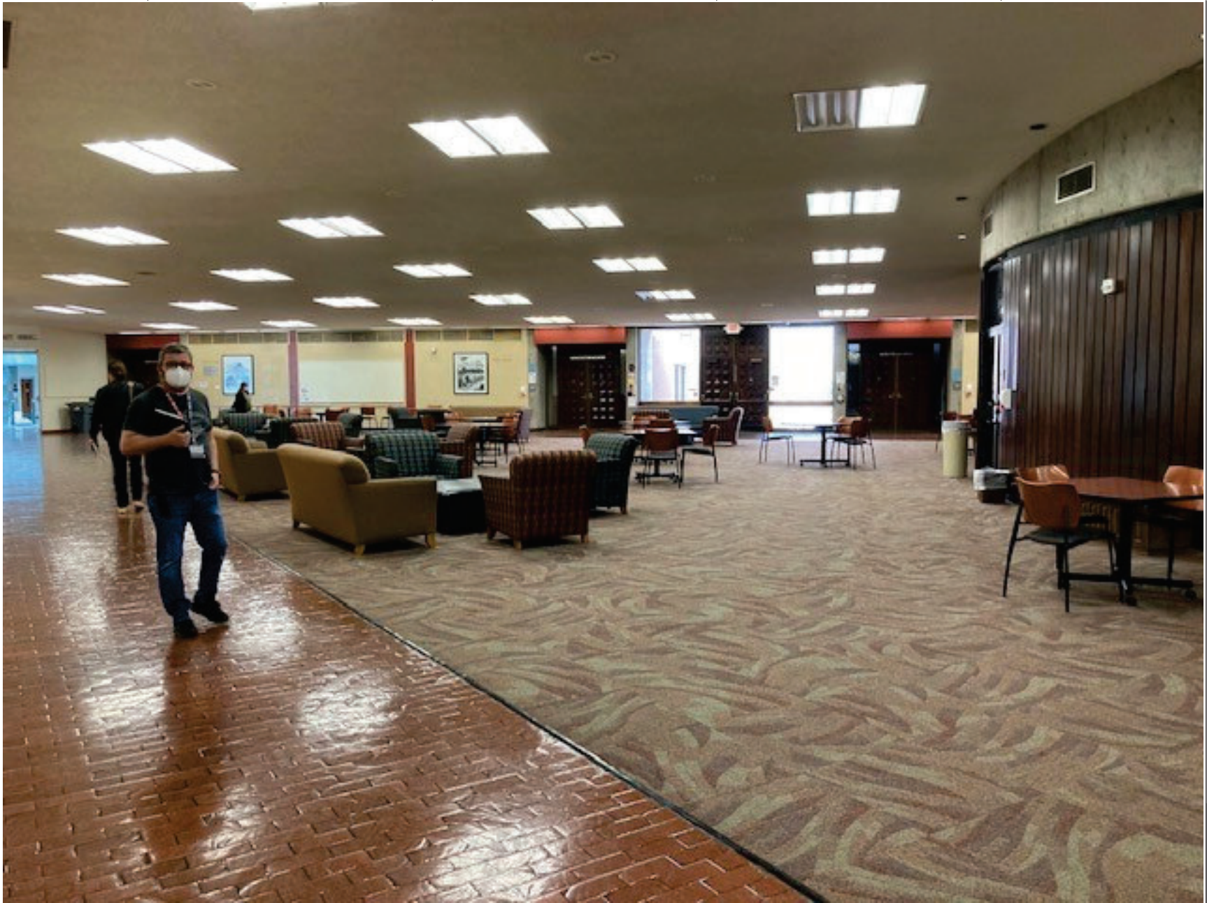
Existing Lobby Finishes with dated carpet and paint scheme. Paneling and doors from original construction in 1969.
