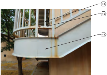
A1 Photo - Rusted Rail NOT TO SCALE
