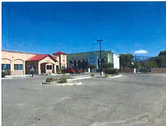
View across parking lot
