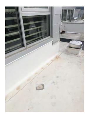
5 Accumulation of Dirt Stepped Metal Flashing
